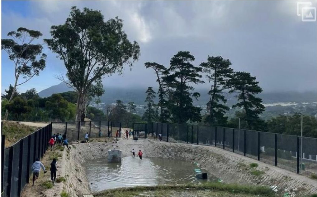
Children are using vandalised stormwater ponds as swimming pools in Hout Bay
