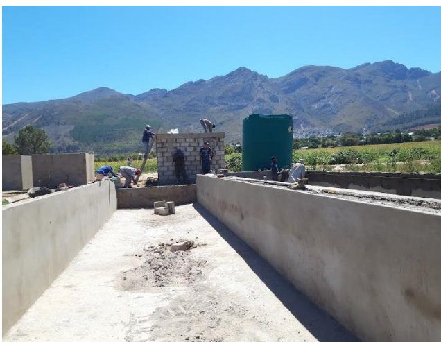
New SMART Cell construction and raising water tanks in 2024
