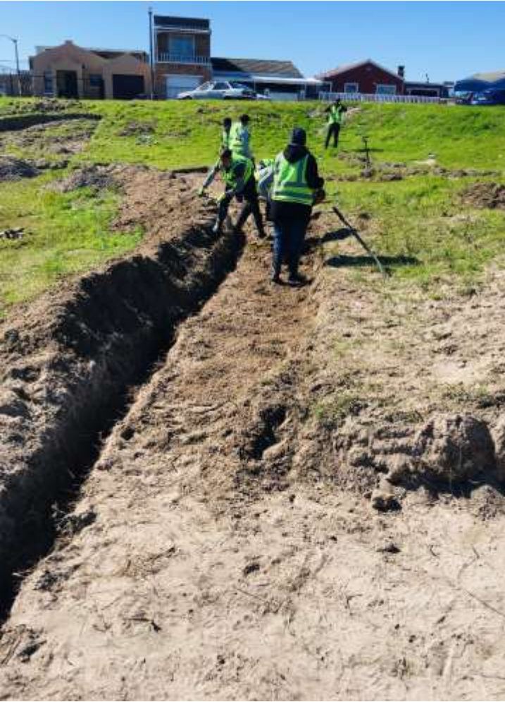
Aug-2021 - Local residents employed to construct infiltration trench and green wall
