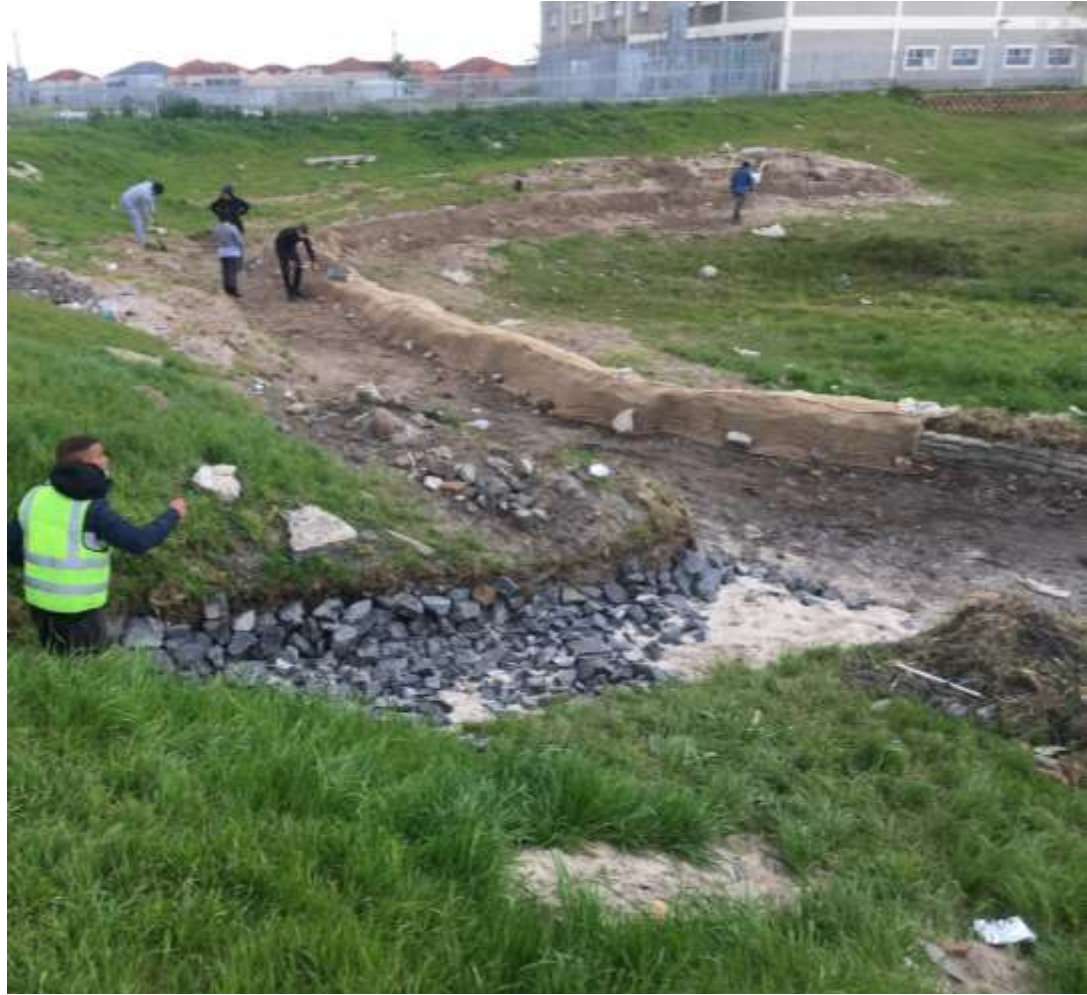
Aug-2021 - Local residents employed to construct infiltration trench and green wall
