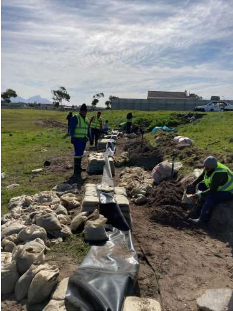
Aug-2021 - Local residents employed to construct infiltration trench and green wall
