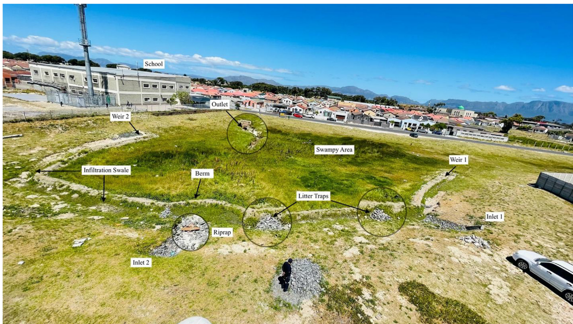
Fig. 3. The stormwater pond retrofit illustrating the different components.
