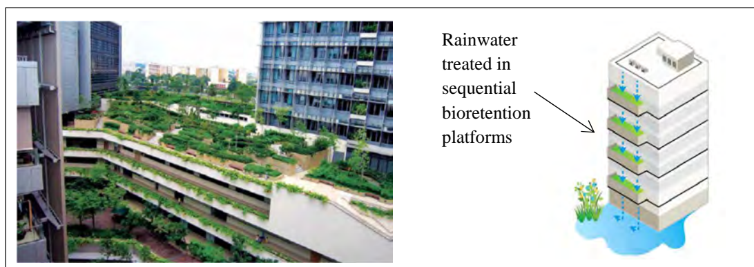
Figure A.7: Sequential vegetated cleaning system – actual (left), conceptual (right) (adapted from PUB, 2011)
